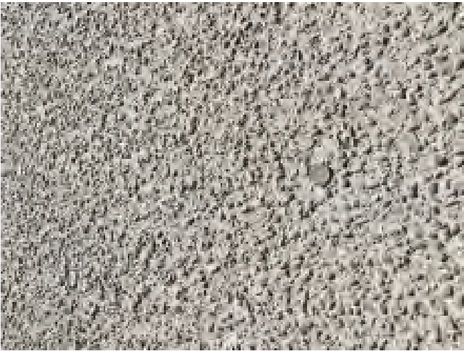
HIGH SEVERITY WEATHERING
